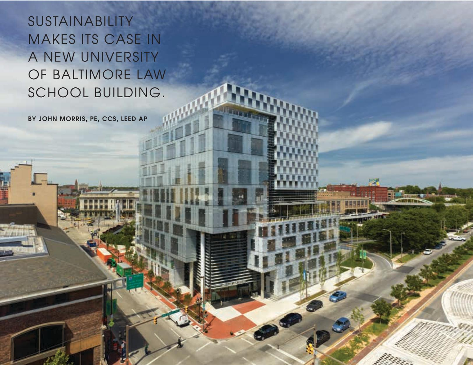
The John and Frances Angelos Law Center is a distinctive new landmark in central Baltimore. The thermal mass of the concrete, 12-story structure is leveraged to reduce heating and cooling loads.
