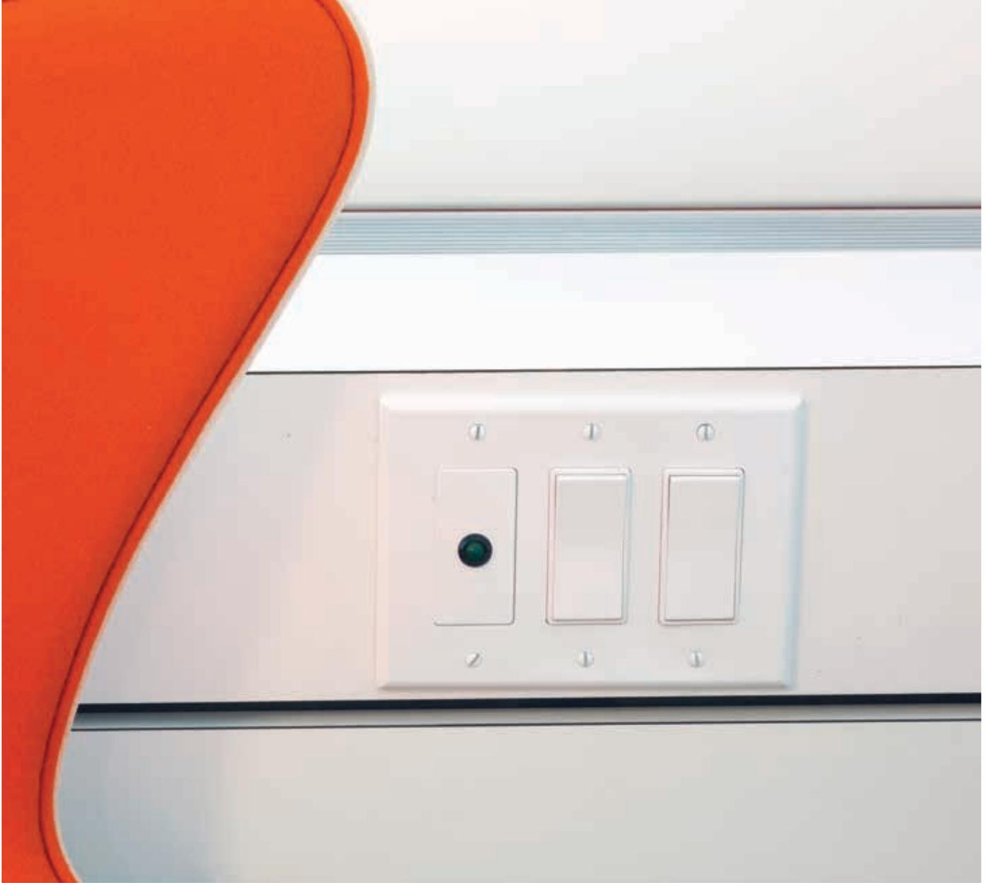
A signal light informs occupants of the option to activate the window and shade-control systems manually. Beneath the control panel, custom millwork houses fin tube heating and wire management.
